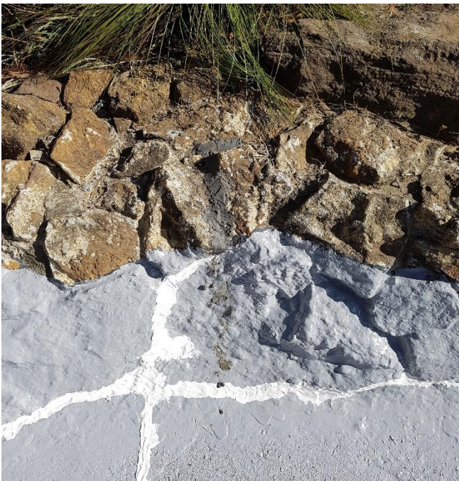
Fig 1.0 Surface Preparation – Pond Surface
