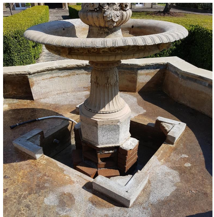
Fig 1.1 Existing surface with active water ingress from ground water
