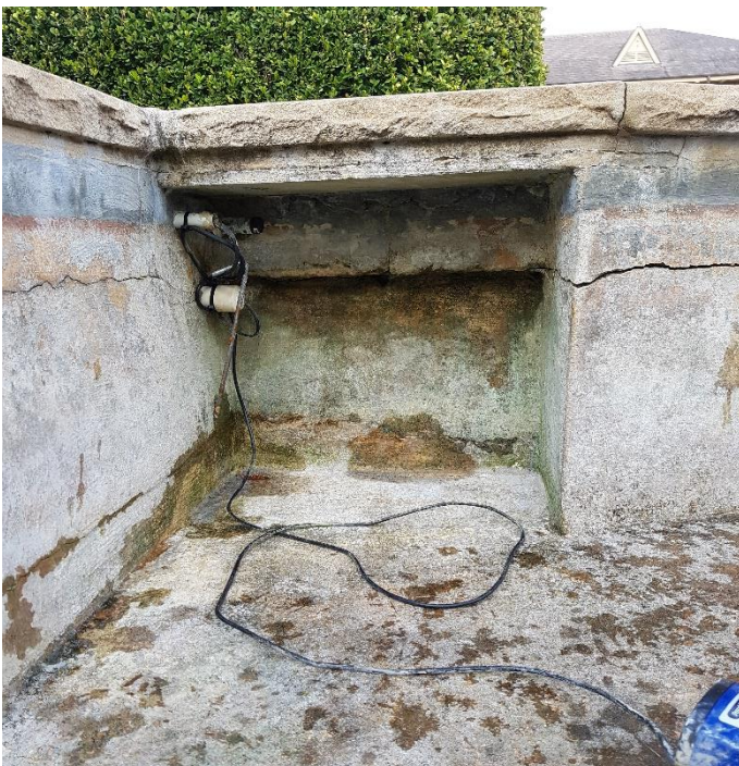
Fig 1.0 Pond in established gardens – ground water following contours of the land and leaking into pond via cracks
