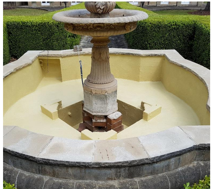
Fig 2.4 Pond Sealer Sandstone application – positive side membrane
