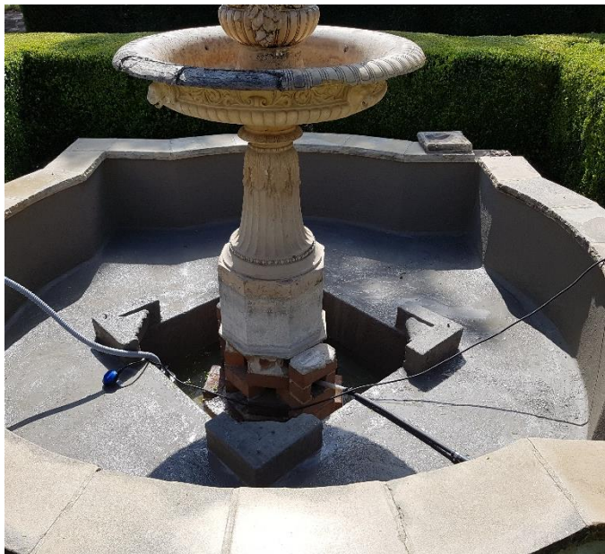
Fig 2.3 Cemproof Flex application – negative side membrane
