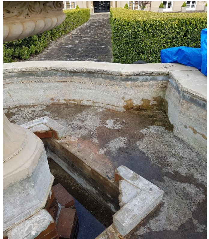
Fig 1.1 Existing surface with active water ingress from ground water
