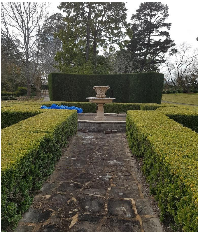
Fig 1.0 Pond in established gardens – ground water following contours of the land and leaking into pond via cracks
