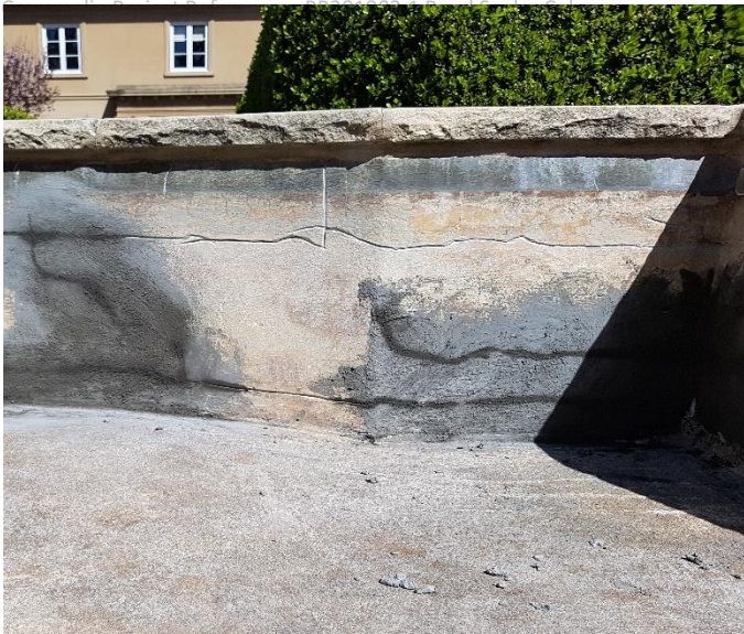
Fig 2.1 Cemproof Plug application – active cracks below ground level
