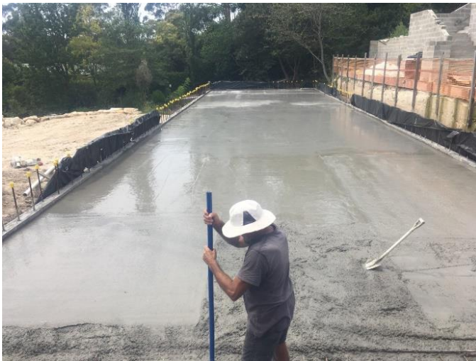
Fig 3.0 Installation of Concrete Tank lid
