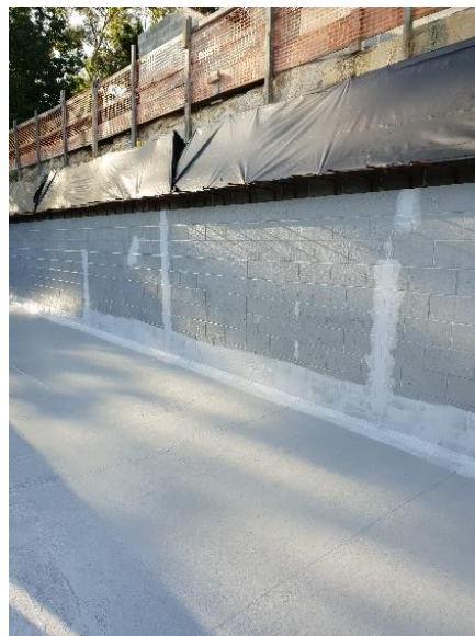
Fig 4.0 Elastoseal TR® / Polyfab crack reinforcement
