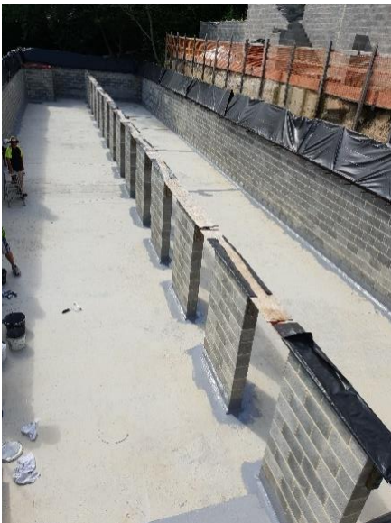
Fig 3.1 Wall / Floor Fillet Preparation
