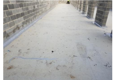
Fig 3.0 Wall / Floor Fillet Preparation
