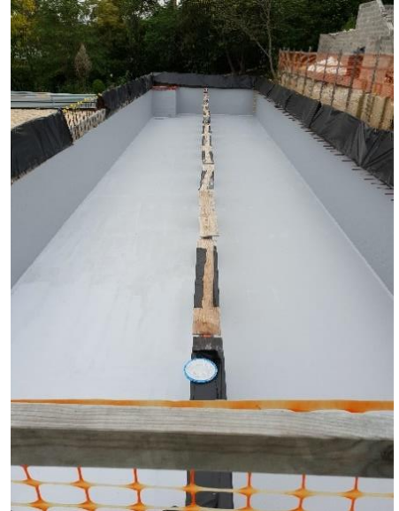
Fig 4.7 Elastoseal TR® Application Completed
