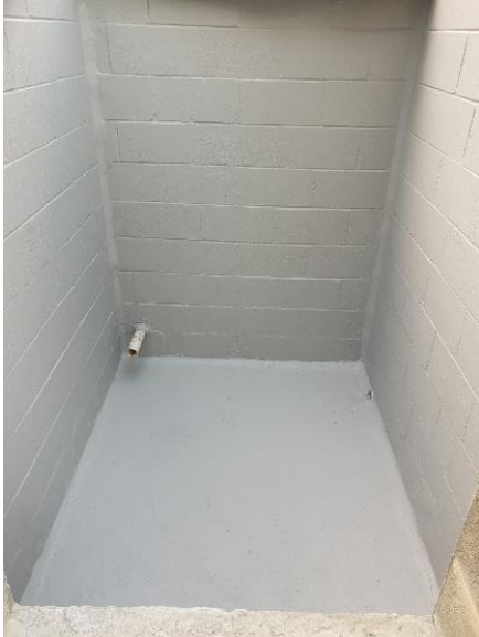
Fig 4.5 Elastoseal TR® Application to Pump Room
