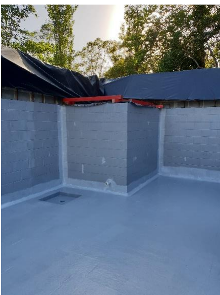
Fig 4.2 Elastoseal TR® Application to Main Tank
