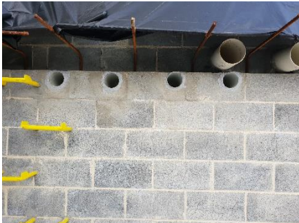
Fig 1.0 Wall Substrate / Inlet Pipes
