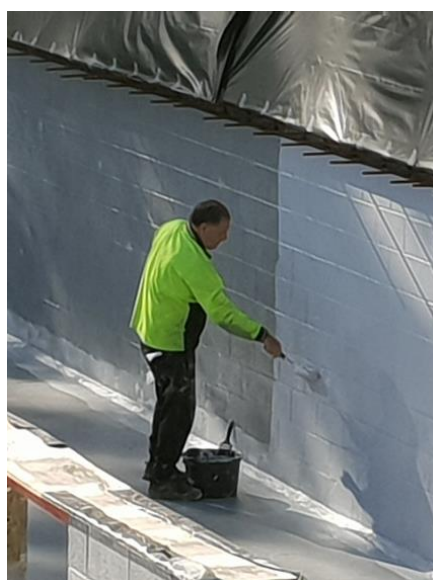
Fig 4.3 Elastoseal TR® Application to Main Tank
