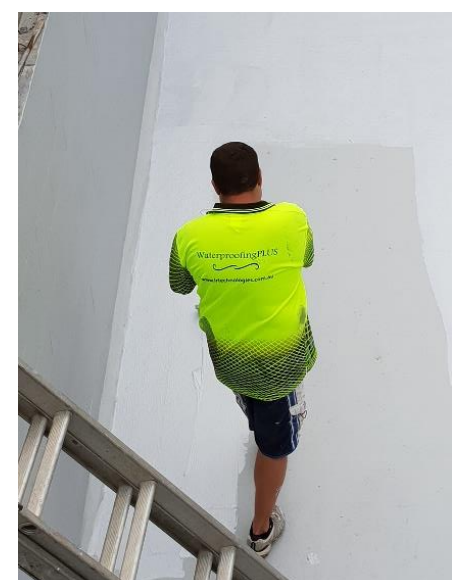
Fig 4.4 Elastoseal TR® Application to Main Tank
